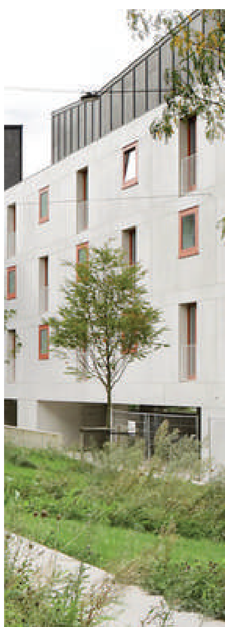
p-garage begane grond
